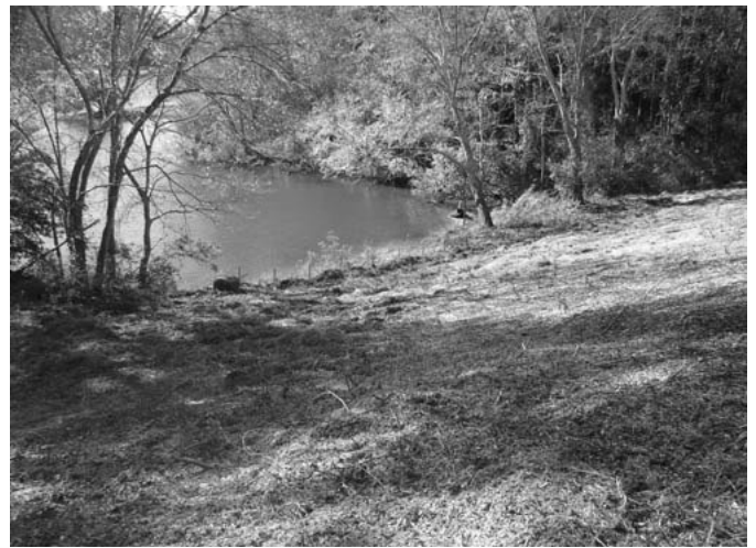
Lower Dam clearing project November 2009
